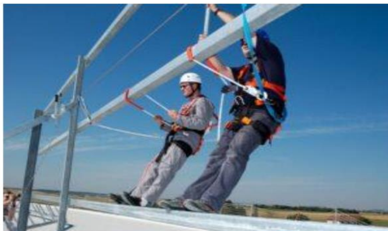
Figure 1. Proper use of protective equipment when working at height
